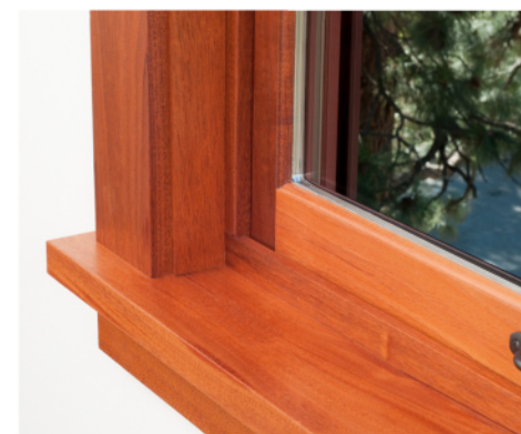
Window sill restoration.
